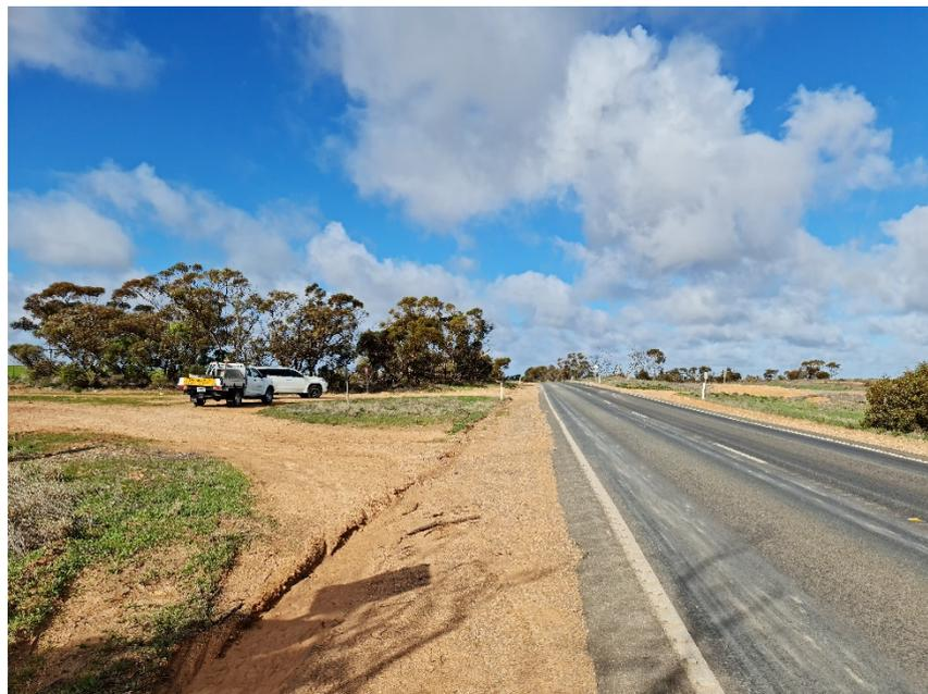
*Picture 5 Condition of exiting table drain at the intersection.*
