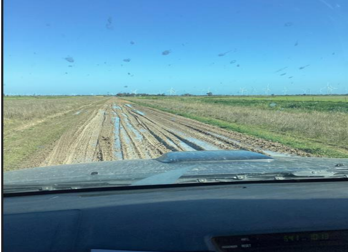
Picture 3 Road condition of Yarriambiack Drive
