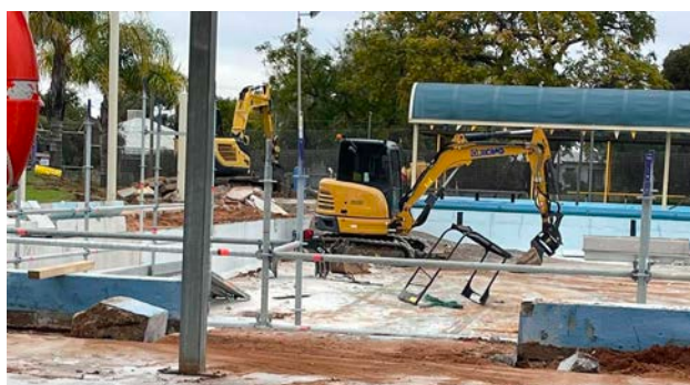
Works happening at Hopetoun Swimming Pool
