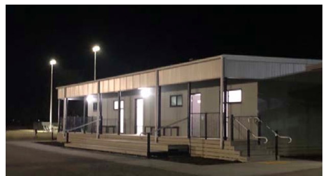
New Netball Changerooms at Minyip for Minyip Murtoa (Burra's) Football Netball Club
