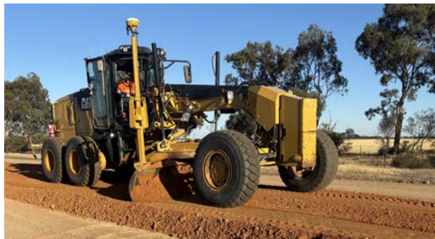
Works carried out on Banyena Pimpinio Road
