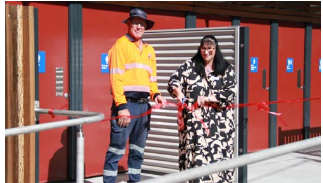
New amenities block with access ramp at Warracknabeal
