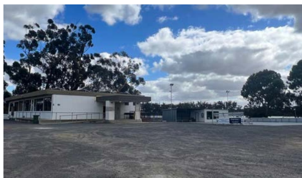
Murtoa Recreation Facilities & Courts
