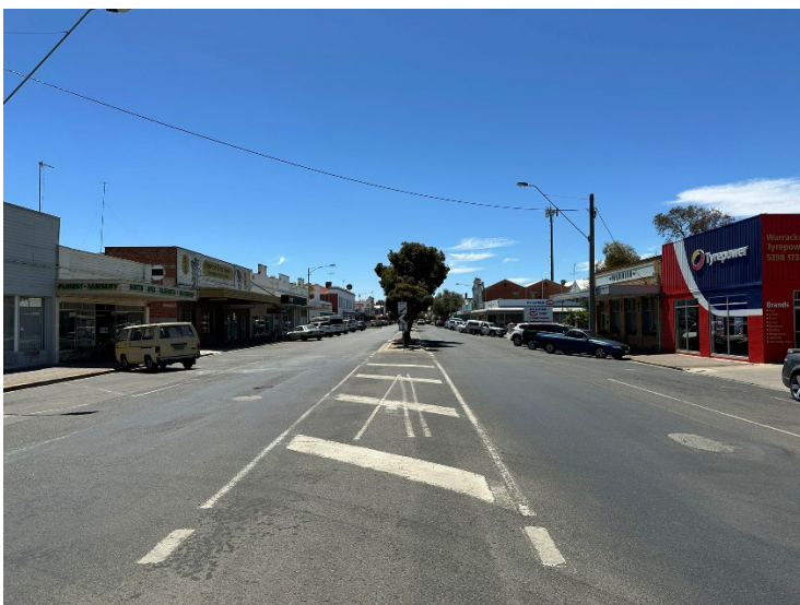
Figure 19: south down Scott Street (centre)
