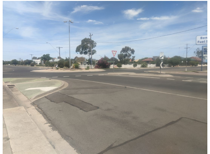
Figure 7: west across Scott and Lyle Street
