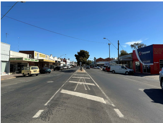
Figure 14: south down Scott Street (centre)
