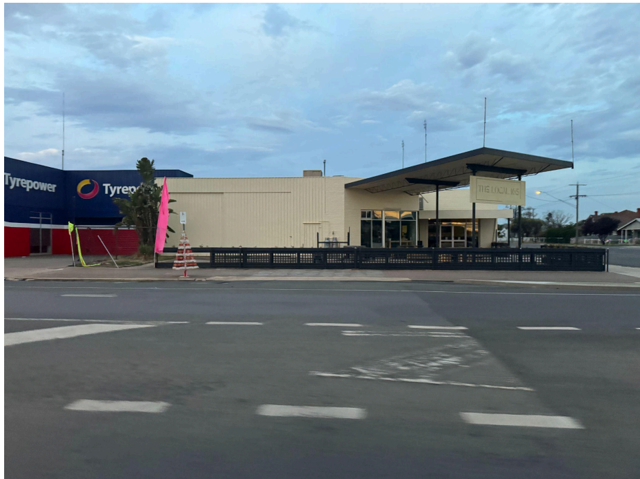
165 - 167 Scott Street, Warracknabeal - Western Elevation
