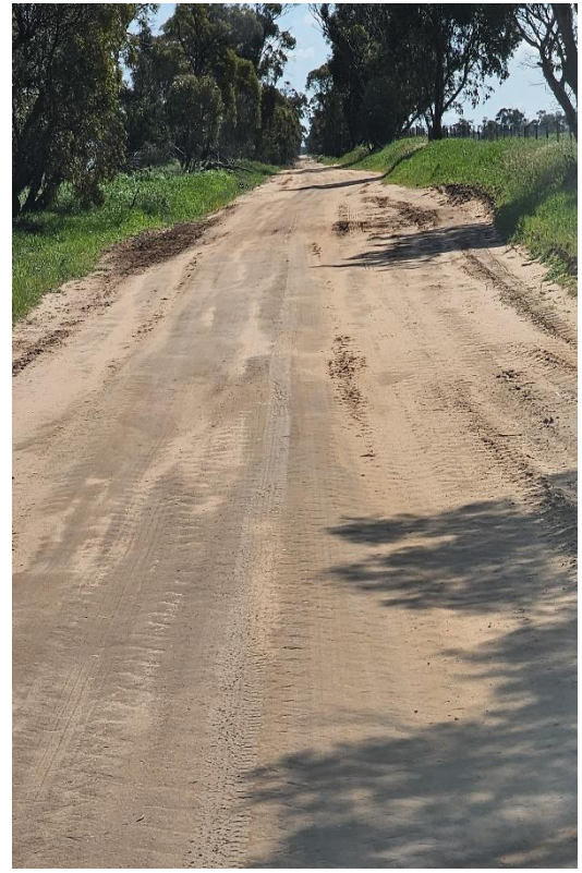
Photo 5 Section of Martins Road where grading required.
