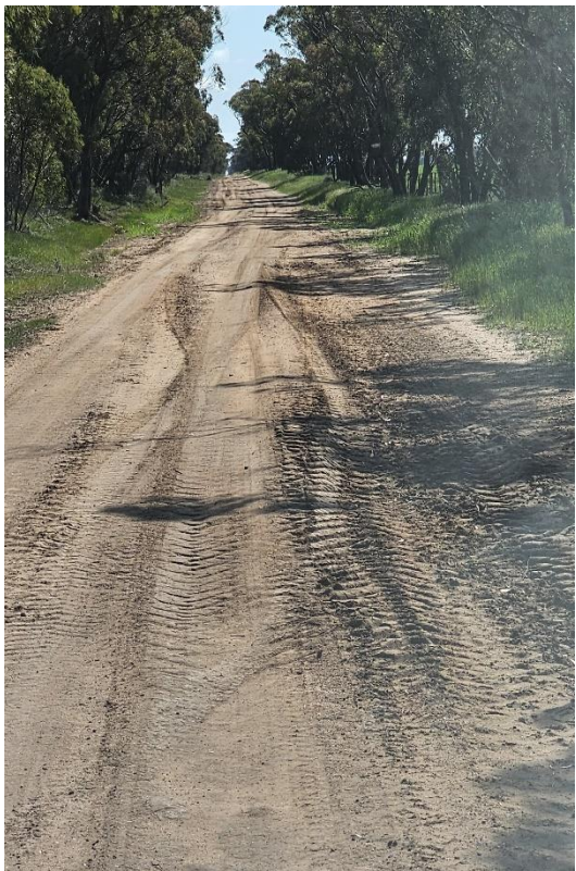
Photo 6 Section of Martins Road where grading required.
