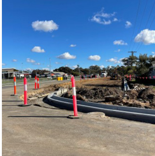
New kerbing in Werrigar St Warracknabeal
