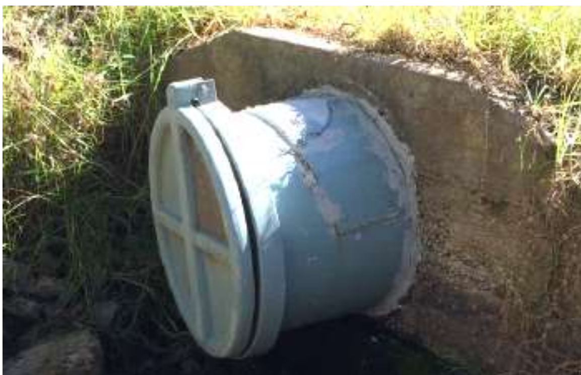
One way flap valve on a stormwater drain at Lyle Street Warracknabeal Weir Pool eastern culverts (Water Technology 2016).
