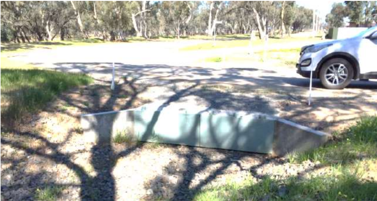
One way culvert flap valves at Asquith Reserve/McIntyre Street Warracknabeal Weir Pool eastern culverts (Water Technology 2016)
