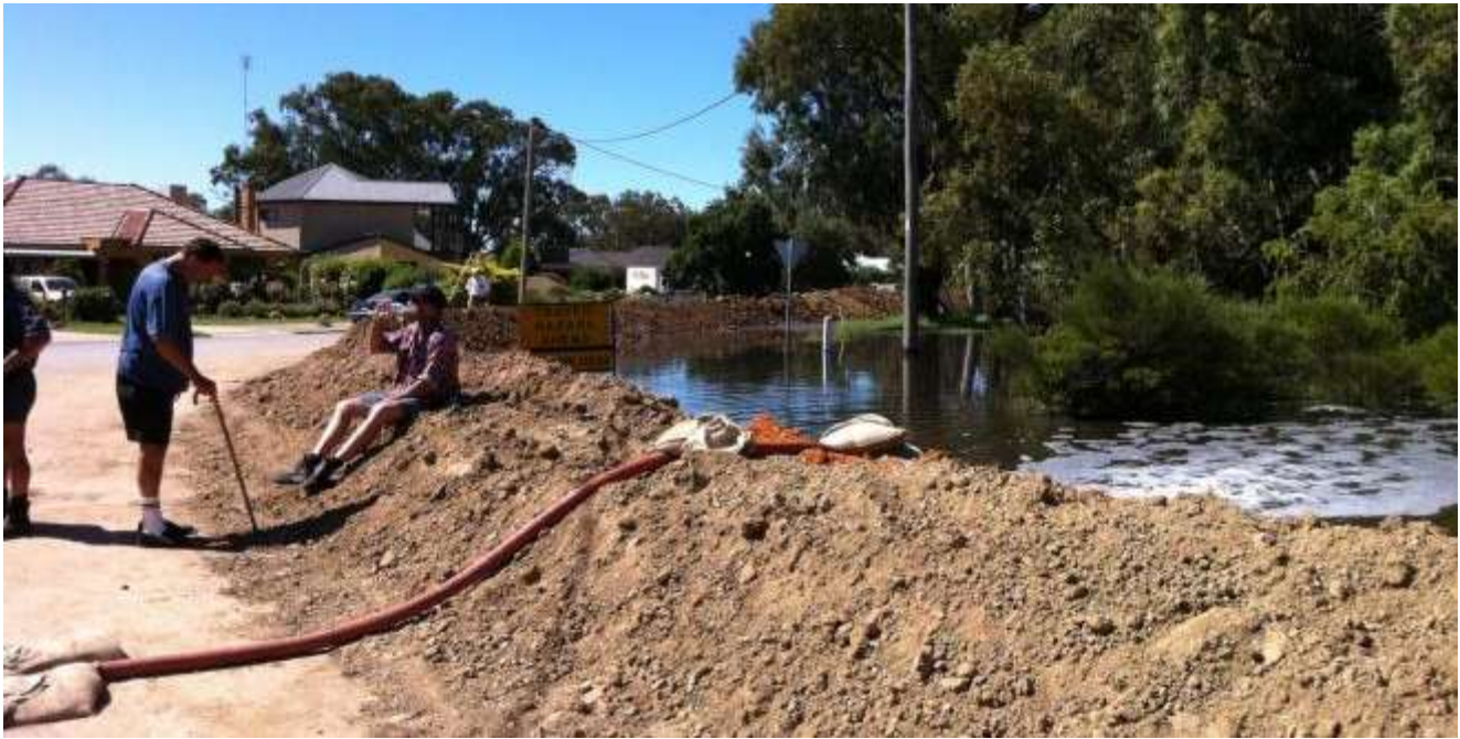
The temporary earthen Warracknabeal Levee constructed during the January 2011 flood event.
