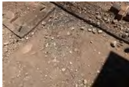
Debris on Ground
