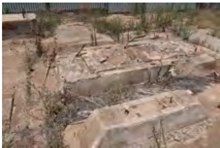
Debris on Ground
