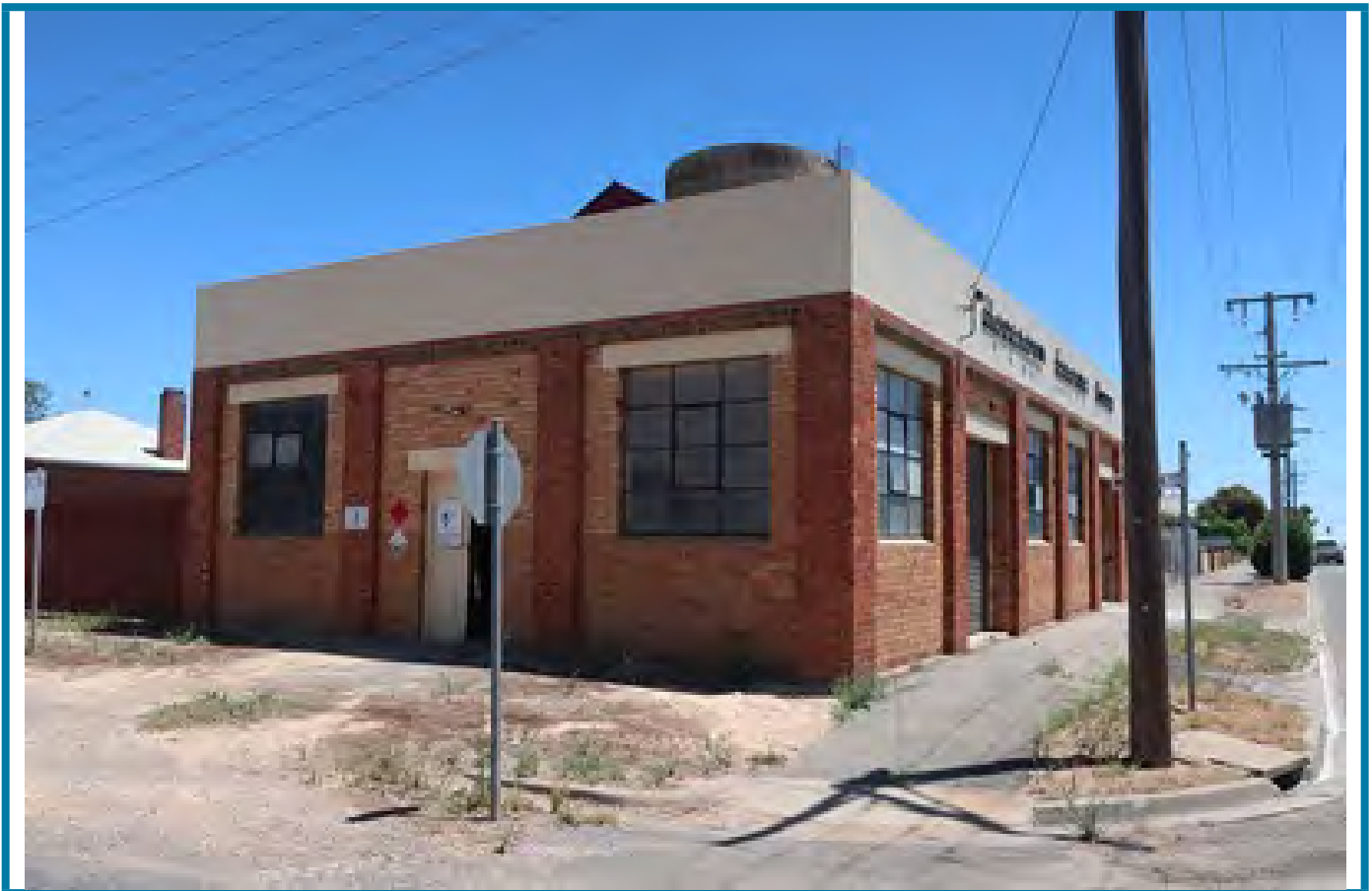
Yarriambiack Shire Council Old Powerhouse (depot) 51 Lascelles Street Hopetoun Vic 3396
