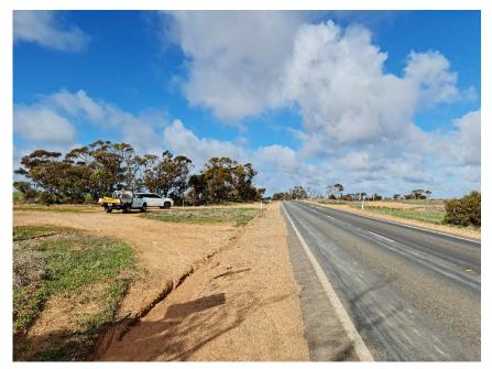
Picture 5 Picture 5 Condition of exiting table drain at the intersection.
