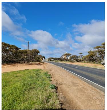
Picture 7 Approach sight distance to the north along Sunraysia Highway from Crook Road exit is restricted by trees.
