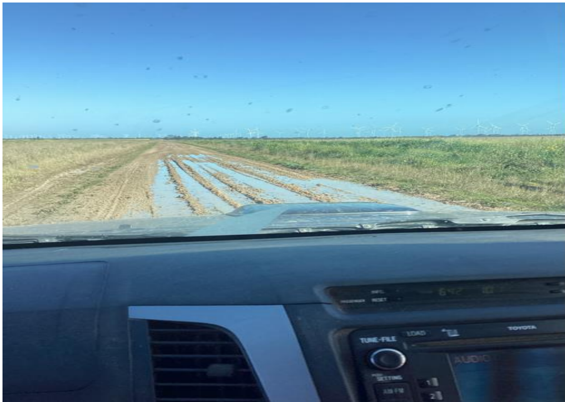
Picture 2 Road condition of Yarriambiack Drive
