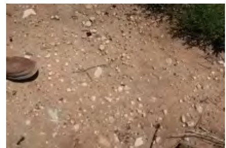
Debris on Surface
