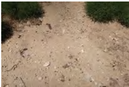
Debris on Surface
