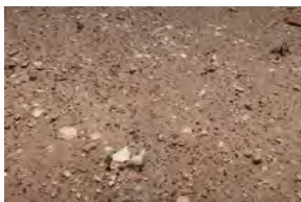
Debris on Surface
