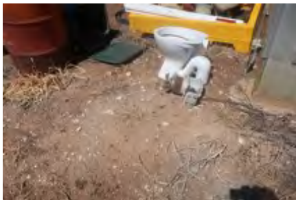
Debris on Surface
