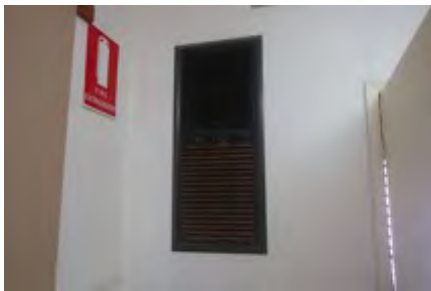
Maintain paint or sealant
