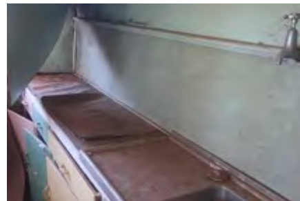
Maintain paint or sealant
