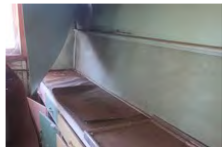
Maintain paint or sealant
