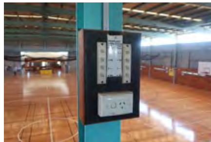
Maintain paint or sealant
