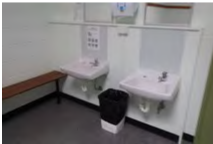
Maintain paint or sealant
