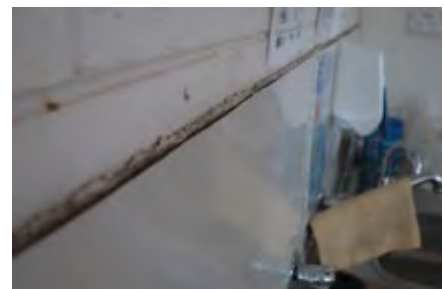
Maintain paint or sealant
