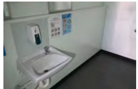
Maintain paint or sealant
