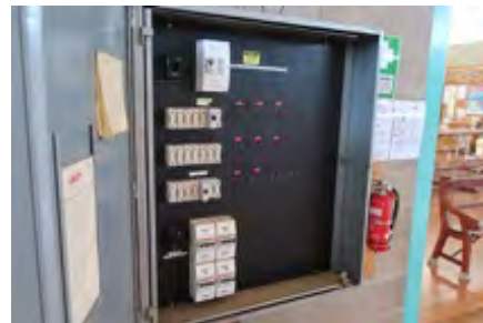
Maintain paint or sealant
