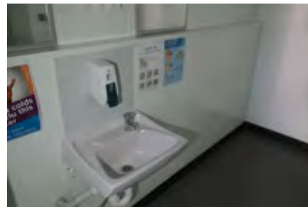
Maintain paint or sealant
