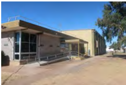
Maintain paint or sealant
