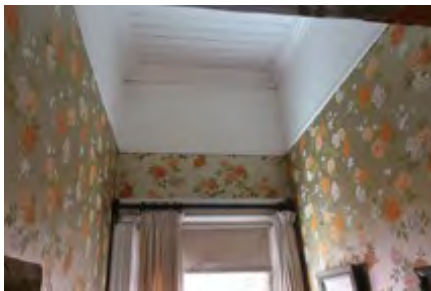
Maintain paint or sealant
