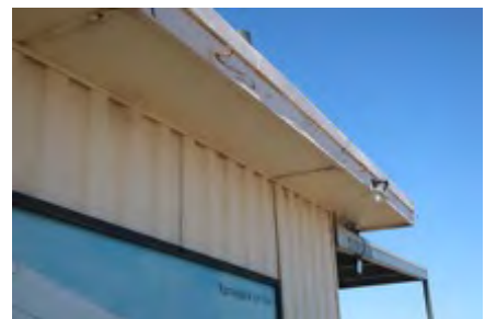
Maintain paint or sealant
