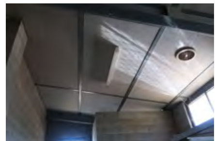
Maintain paint or sealant
