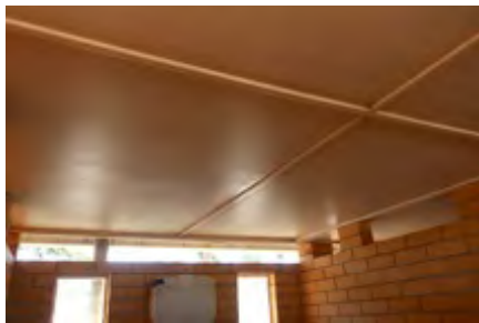
Maintain paint or sealant
