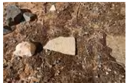
Debris on Surface
