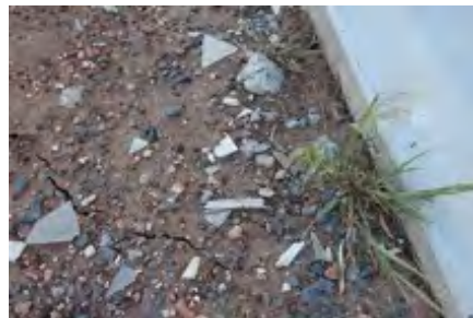
Debris on Surface
