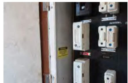
Maintain paint or sealant
