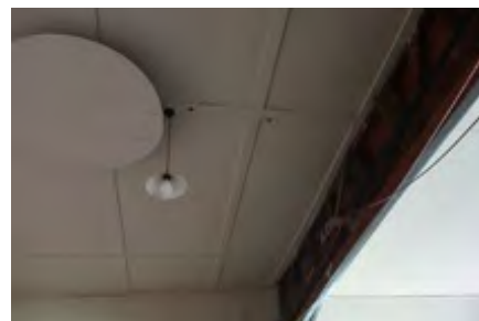
Maintain paint or sealant
