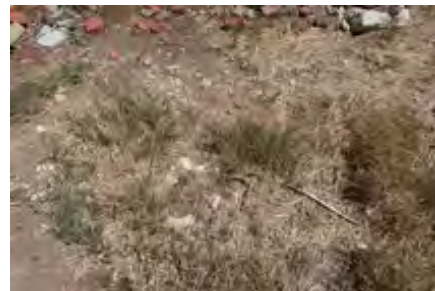
Debris on Surface
