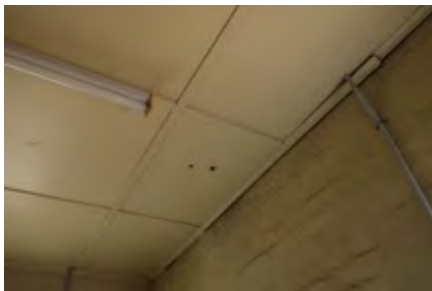
Maintain paint or sealant
