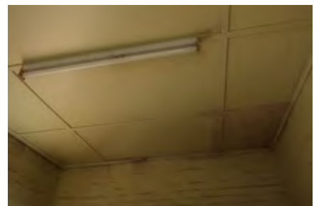
Maintain paint or sealant
