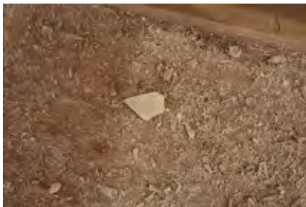
Debris on Surface
