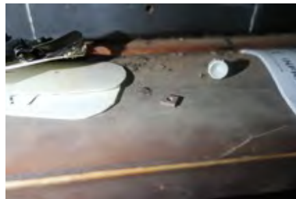
Debris on Surface
