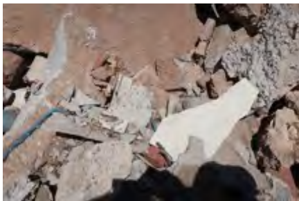
Debris in Tip Pile
