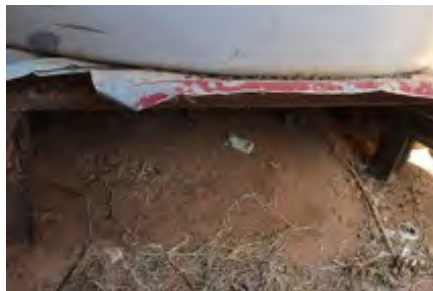
Debris on Ground
