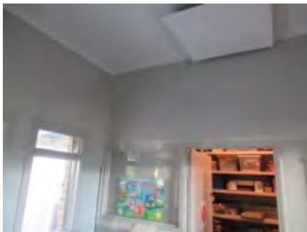
Maintain paint or sealant
