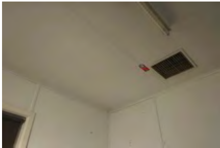
Maintain paint or sealant
