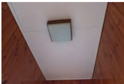
Maintain paint or sealant
