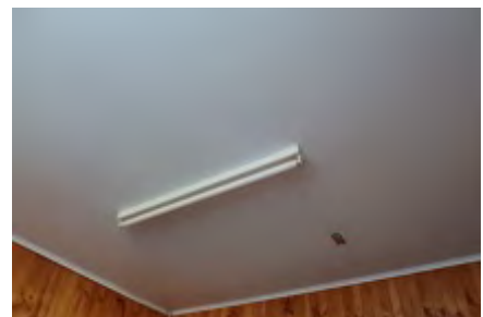
Maintain paint or sealant
