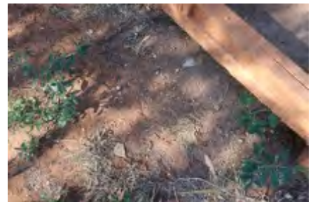
Debris on Ground
